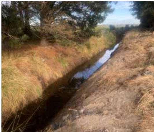
Steep banks without vegetation cover are a source of fine sediment to the drainage waterways.
