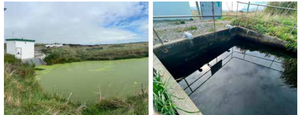
The Osbornes pump station is not a fish-friendly design, nor does it have a bypass channel. An upstream inlet screen and downstream flap gate were installed as a condition of the current consent to impede the access of fish to the pump station.
