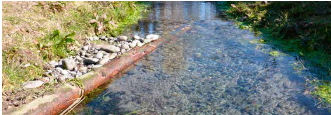
Log vanes are typically installed pointing upstream, and can be used in both small and large channels. They are used to vary instream habitat while also promoting bank stability through the accumulation of sediment. However, with the low water velocity of the Osbornes catchment they might not realise their full potential of creating varied water velocity and stable scour pools.
