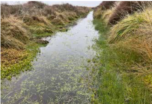
The channel downstream of the pump station alternates between raupō wetland and open water. With a very low gradient, water velocity remains very slow.
