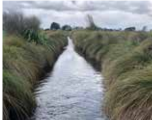
The flat area of water in this channel is a sediment trap location. When the trap is nearly full, a digger can reach over the fence and planting to remove sediment.
