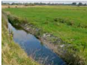
An inline sediment trap may simply be a widened and deepened area of channel, where the flow is slower and encourages the deposition of fine sediment. However, we are recommending a more hard-edged solution, to enable easier access for maintenance.
