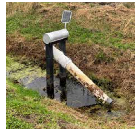
Water level controls can be used to better manage soil moisture levels in dry summer periods. Automated or semi-automated control can improve easy management of the structure.
