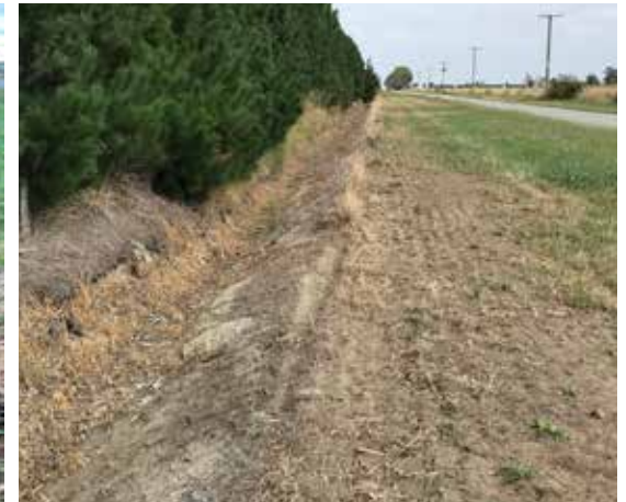
Banks that are regularly sprayed are an ongoing source of sediment to the drainage channel.
