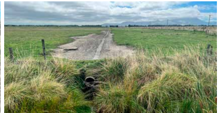
Ephemeral drainage waterways that are dry most of the time become sources of sediment during rainfall as they channel overland runoff to downstream waterways.
