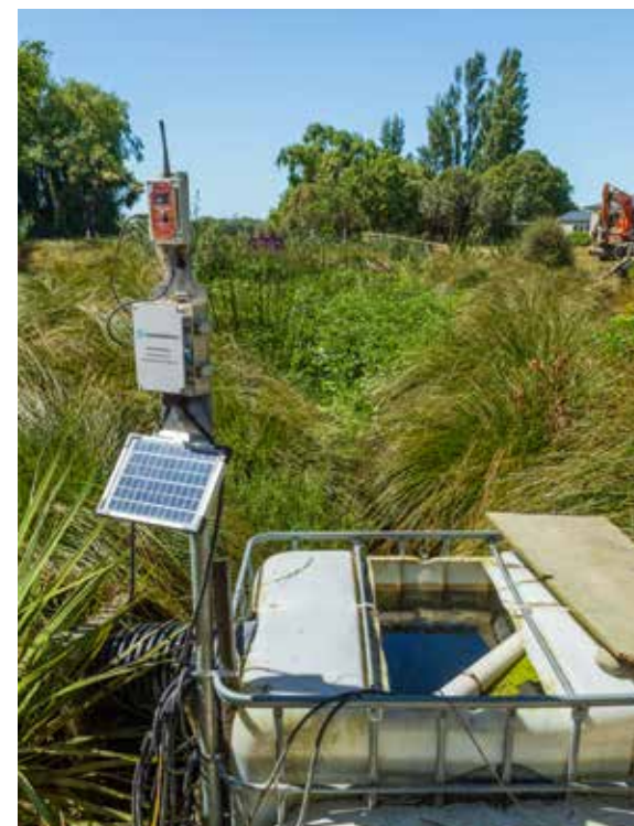
A small-scale off-channel wetland constructed with multiple cells and a control structure to allow for water quality testing and flow control.
