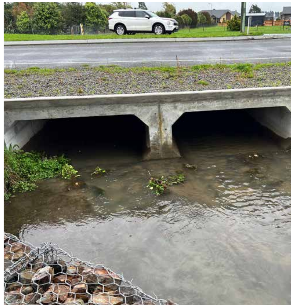
Example of a more suitably sized culvert in the Leeston rated catchment.
