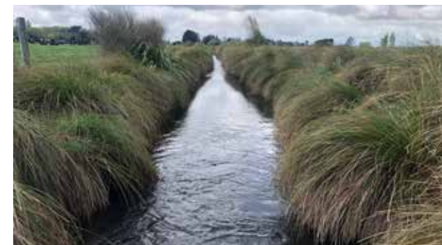
The flat area of water in this channel is a sediment trap location. When the trap is nearly full, a digger can reach over the fence and planting to remove sediment.
