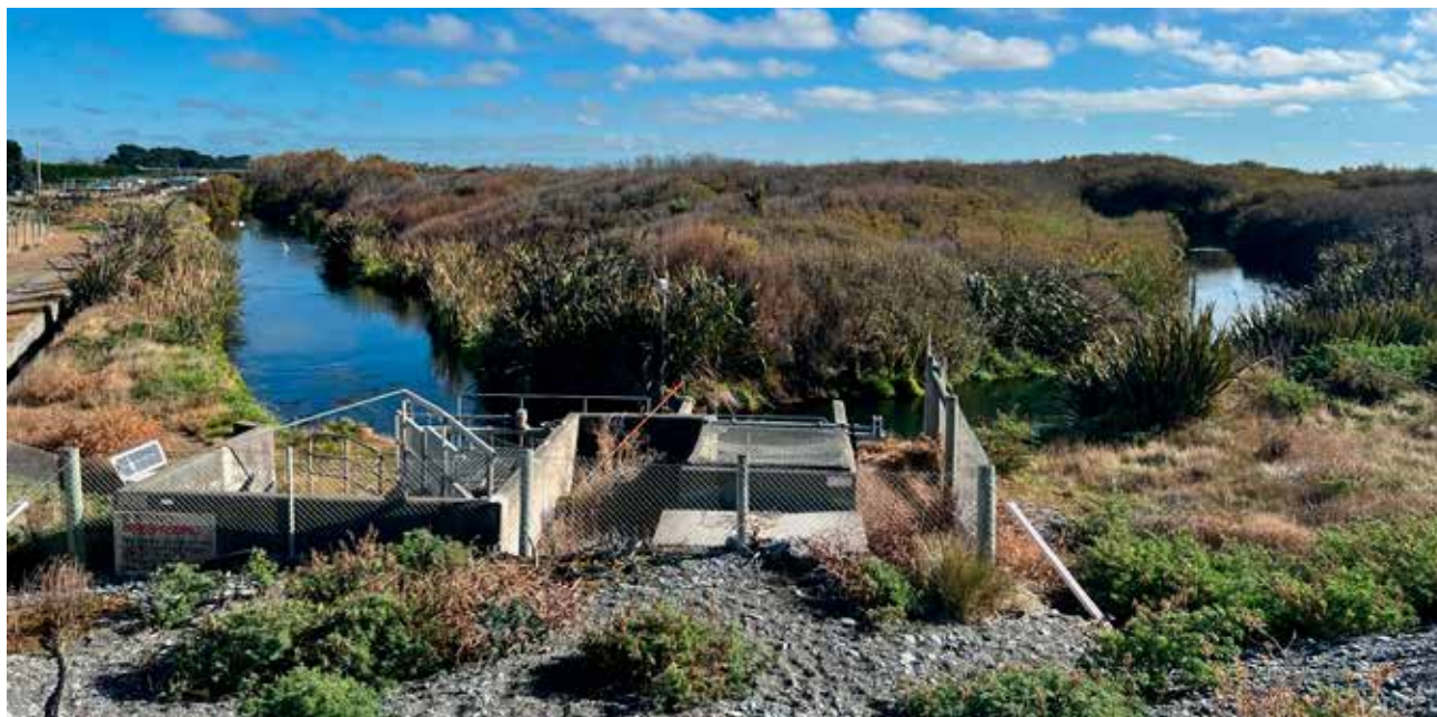
Piped channel outlet to the coast, Taumutu rated catchment.
