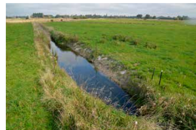
An inline sediment trap may simply be a widened and deepened area of channel, where the flow is slower and encourages the deposition of fine sediment. However, we are recommending a more hard-edged solution, to enable easier access for maintenance. Image source: Robin Smith, DOC
